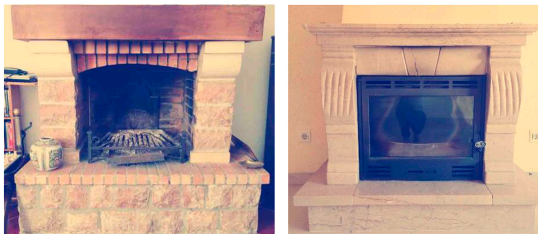
Figure 2. Appliances used for biomass burning include (left) an open fireplace located in the living room of dwelling 2 and (right) a closed fireplace (insert) located in the living room of dwelling 3.
