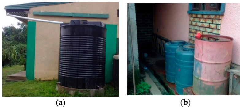
Figure 4. Illustrates the difference between formal and informal rainwater harvesting systems. (a) Formal harvesting systems; (b) Informal harvesting systems.
