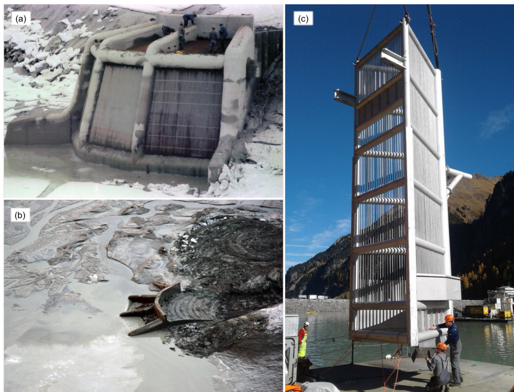
Figure 1. Archive picture of the lower intake structure (a)—situation end of 2015 with the increase sediment level (b)—final works on one trash rack structure (intake tower) near the installation location (c)—(TIWAG).
