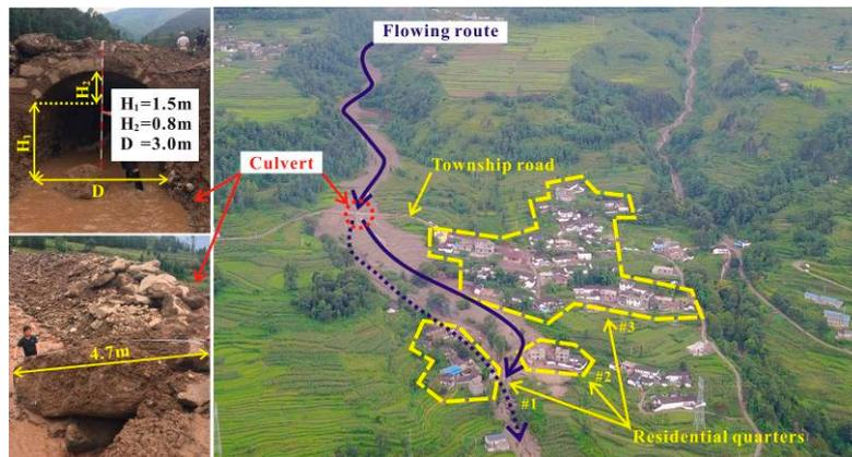
**Figure 6.** Route diversion of the debris flow after the arc culvert of the township road in the inundated or runout area with morphological observation of the cleared arc culvert of the township road and the great stone block in the arc culvert after cleaning (all photos were shot on 9 August 2017).
