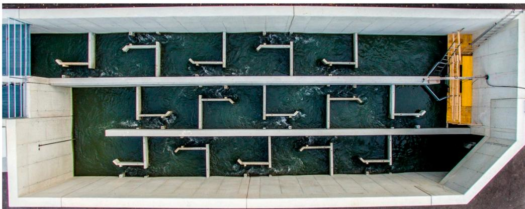
**Figure 2.** Meandering stream course in the *enature*® fish pass, with multiple structured slots arranged in an alternating manner.
