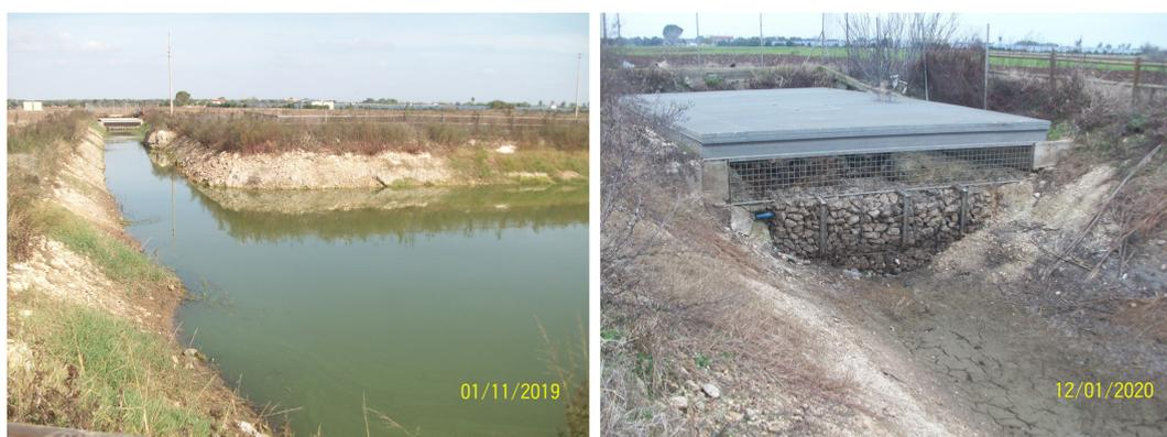
**Figure 8.** Left: the final course of the new channel in the beginning of November 2019; the hydrometric level was at a mean height, despite only 115 mm of rain in the previous four months; right: the entrance of *Vora Manieri* hole in the middle of January 2020; the brownish mud that covers the channel bed could cause clogging processes in the swallow hole.
