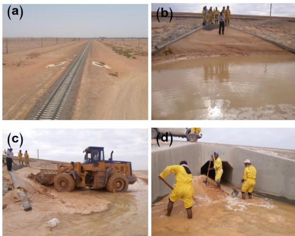
Figure 16. (a) Part of the Al-Shamal train pathway; (b) the existing structures under the train pathway which are blocked by Wadi Bayer floodwater sediments in front of the train pathway; and (c,d) the process of removing sediment from under the Al-Shamal train pathway.
