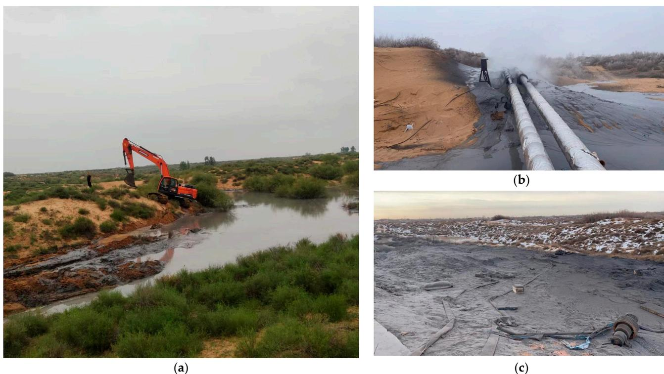
**Figure 1.** (a) River filling caused by grout ground leakage. (b) Grout flow back in borehole. (c) Grout spread on the ground surface.
