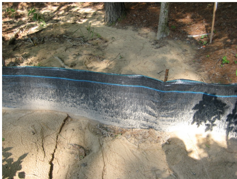
Figure 8. Silt fence installed below the natural gas well pad at F1 illustrating the ineffectiveness of this sediment control technique due to poor installation and large sediment volumes eroded at the Alto Experimental Watersheds in Texas, USA.
