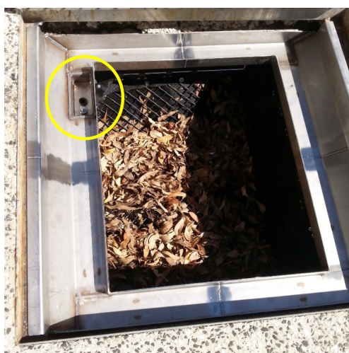
Figure 5. StormSack sample collection photograph (inlet circled).
