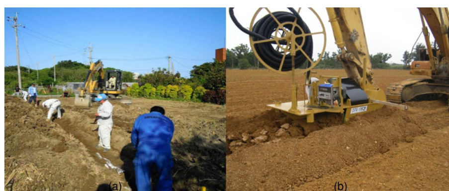
Figure 9. Installation of OPSIS lines (a) Manually laying out lines, (b) Use of machine to lay out lines.
