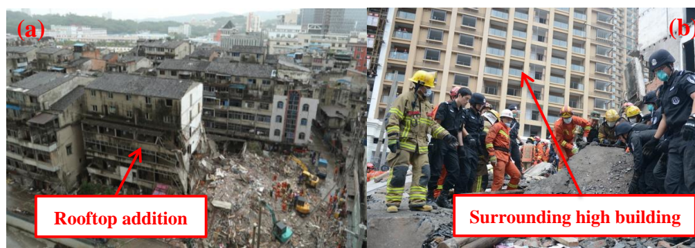
Figure 4. Scene of collapsed incident on 10 October 2016: (a) rooftop addition of collapsed building; (b) surrounding high building at collapsed site.
