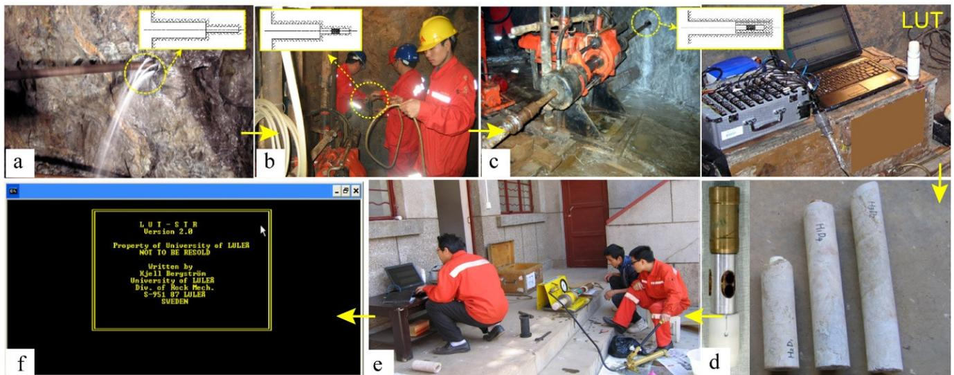
**Figure 10.** Stress relief process: (a) drilling and cleaning; (b) installing strain gauge probe; (c) stress relief and data acquisition; (d) obtaining core tube; (e) confining pressure calibration; (f) in situ stress calculation.
