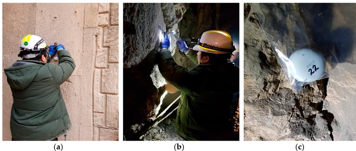
**Figure 4.** Installing Bluetooth beacons (a) in the portal of the mine and (b) in the underground mine; (c) Bluetooth beacon with minor ID 22.
