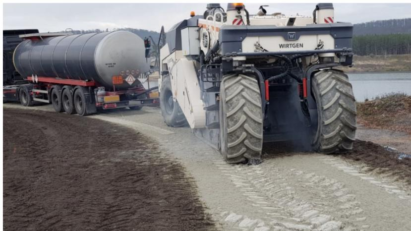
**Figure 4.** Preparation of the recycled mixture under field conditions using the "in situ" method [P. Buczyński].
