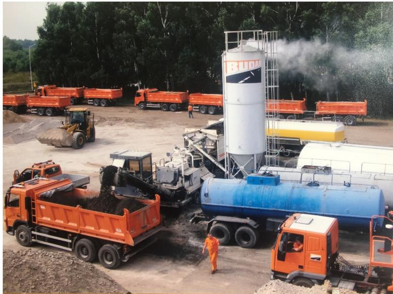
**Figure 2.** Performing of the MCE mixture using the “in-place” method. [J. Krasowski].
