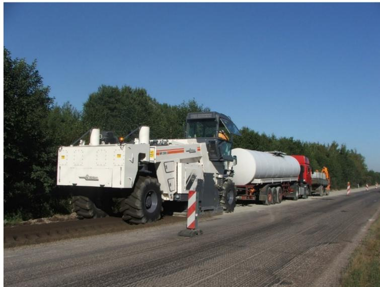
**Figure 1.** Manufacturing of the bitumen emulsion (MCE) mixture using the “in-place” method. [J. Krasowski].
