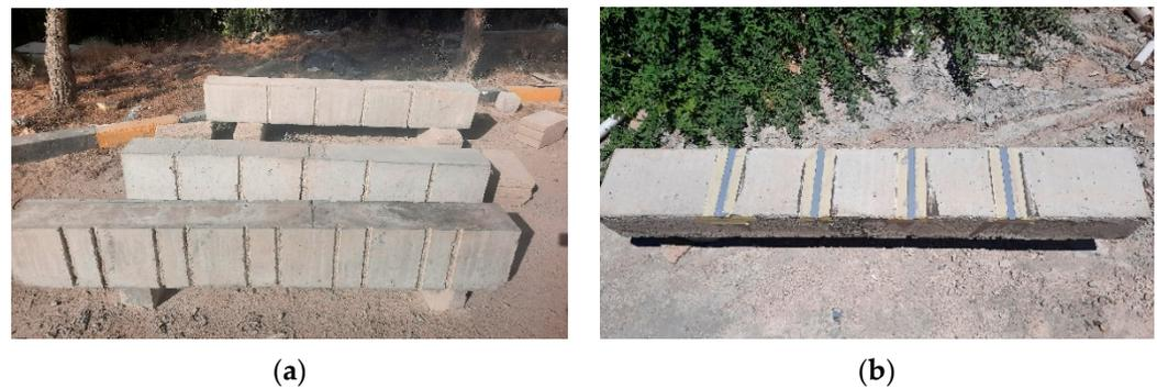
**Figure 4.** NSM-CFRP installation: (a) preparation of groove and (b) NSM-CFRP installation.
