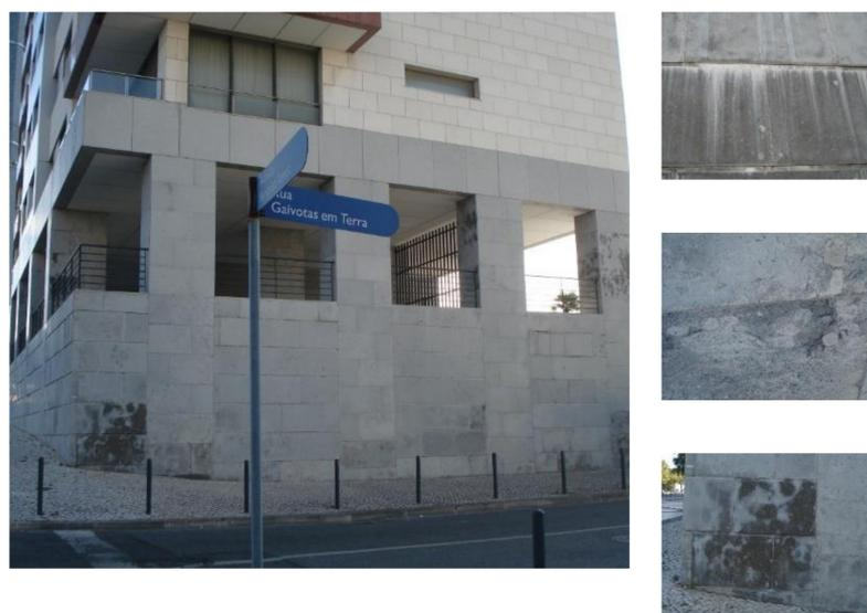
Figure 2. Second case study: natural stone cladding.
