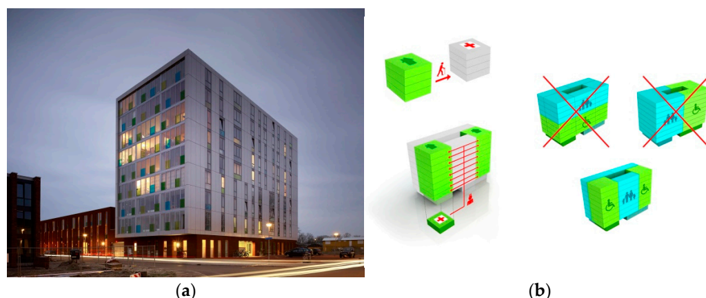
Figure 4. Hybrid apartment tower in Groningen, Netherlands (a) and diagram of integration of health, care, and housing within the apartment block (b). Photo: Christian Richter. Drawings: Casanova + Hernandez Arquitectos.
