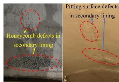
Figure 3. Tunnel second lining defect.
