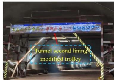
**Figure 4.** Tunnel second lining modified trolley.
