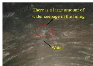
Figure 1. Seepage and leakage of tunnel lining.
