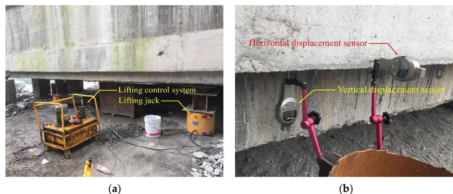
**Figure 11.** (a) Lifting system; (b) displacement sensors.
