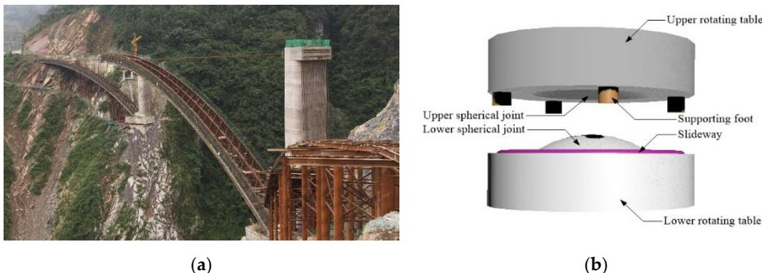
**Figure 1.** (a) Rotating system and rotating construction process; (b) spherical joint.
