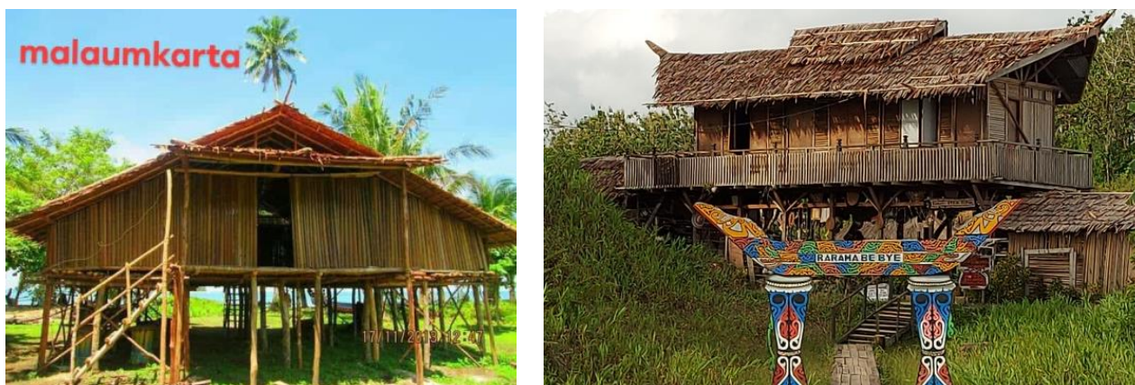
Figure 1. Traditional building design using sago midrib for the house's roof.
