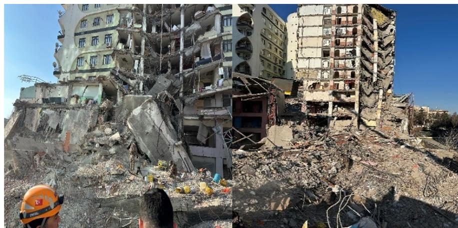
**Figure 6.** Collapsed buildings in Diyarbakır.
