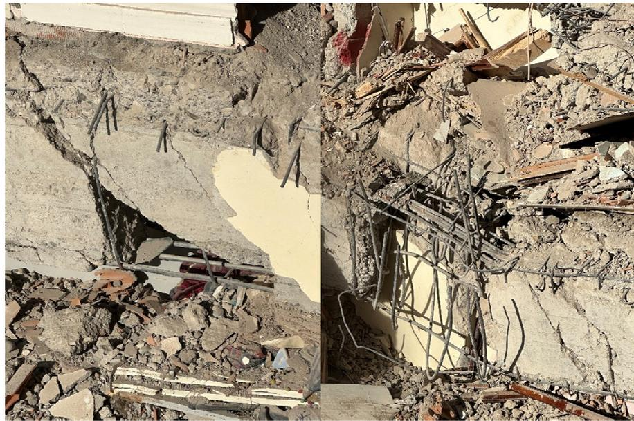
Figure 7. Shear damage of the beam and inappropriate stirrups.
