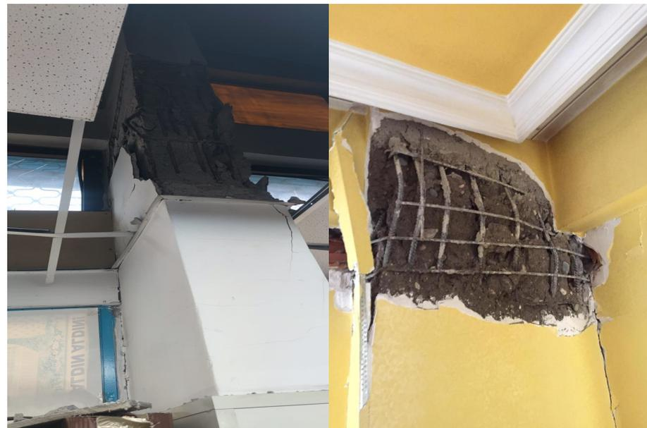
**Figure 10.** Damage to the short column and shear wall with poor concrete.
