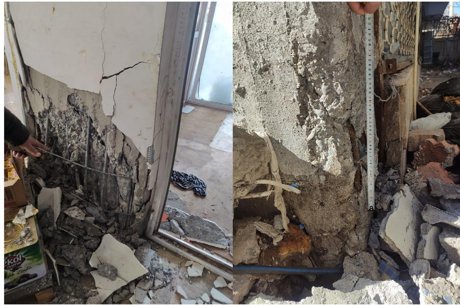
**Figure 9.** Extensively damaged columns.
