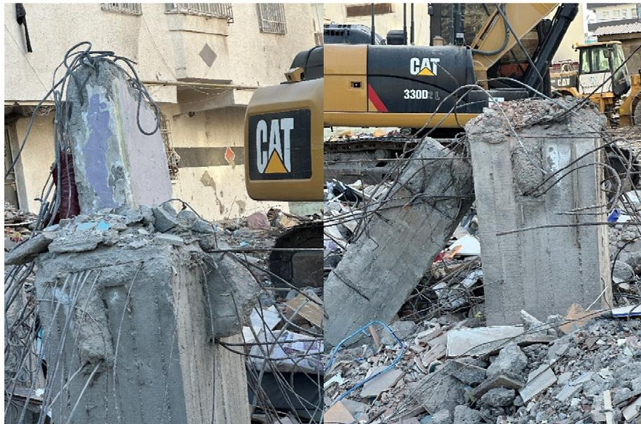
Figure 8. Retrofitting of the ground floor only and the failure of the old column.
