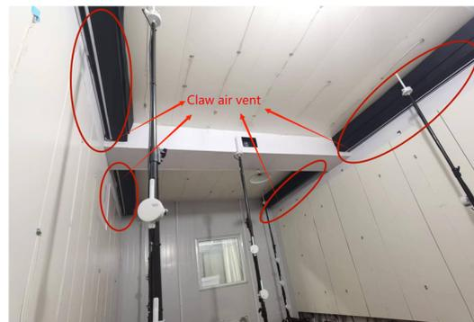
**Figure 3.** Physical diagram of symmetric-wall radiation combined with adherent-jet air conditioning system.
