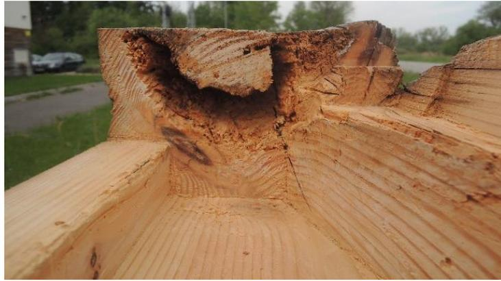
**Figure 25.** Detail of a hole left in the end of the damaged beam after the cleaning.
