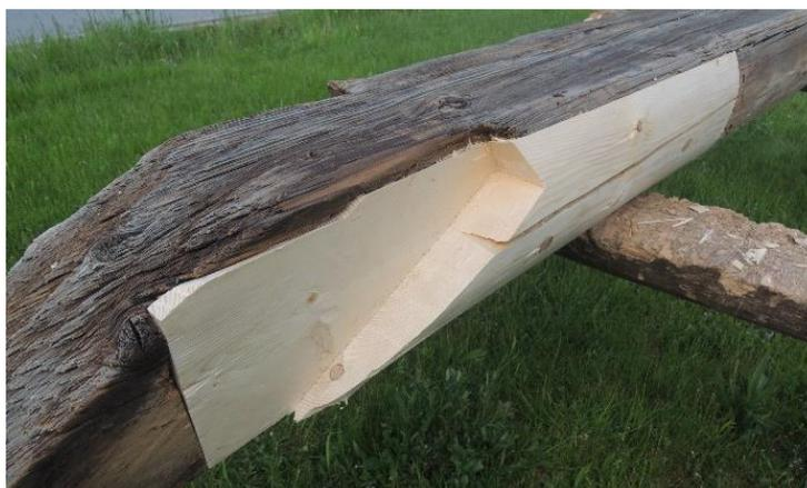
**Figure 31.** Dovetail joint of the damaged timber beam (I2) after the repair.
