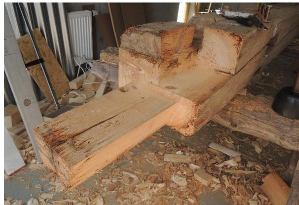
**Figure 6.** Gradual removal of the damaged wood at the beam bottom (after cleaning).
