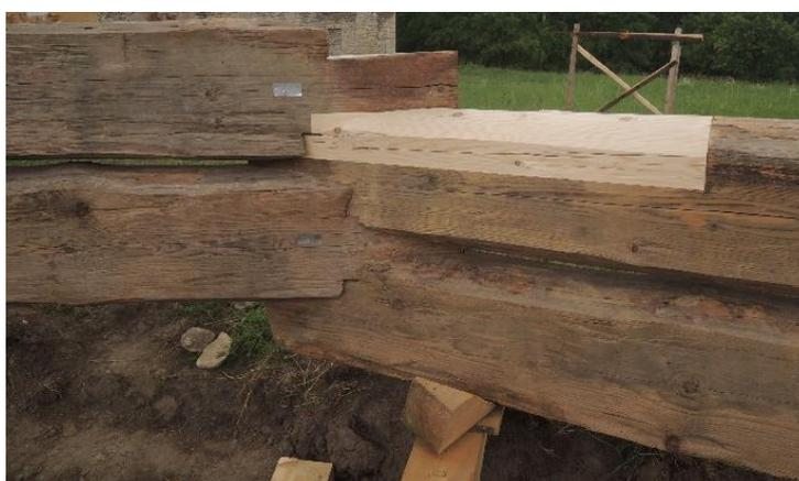
**Figure 32.** The repaired beam put back to its original place in the barn timber wall (inside view).
