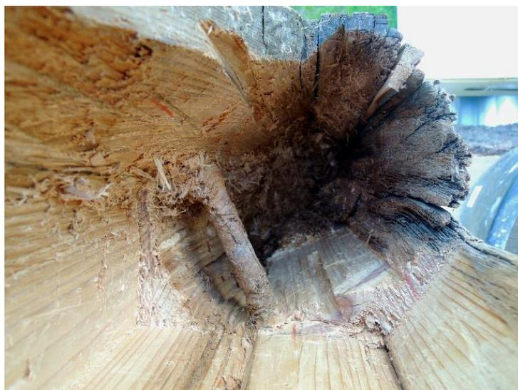
**Figure 16.** Detail of the cleaned hole in the central part of the beam, including the grooves for the rear insert.
