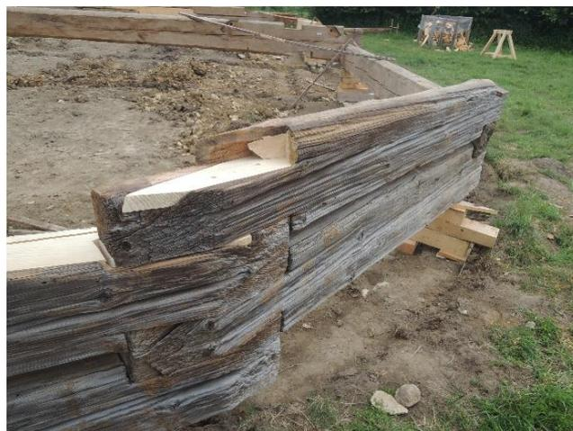
**Figure 20.** The repaired beam put back to its original place in the barn timber wall.
