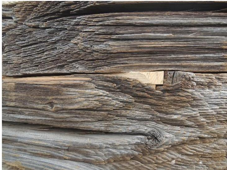
**Figure 26.** The repaired beam put back to its original place in the barn timber wall (outside view).
