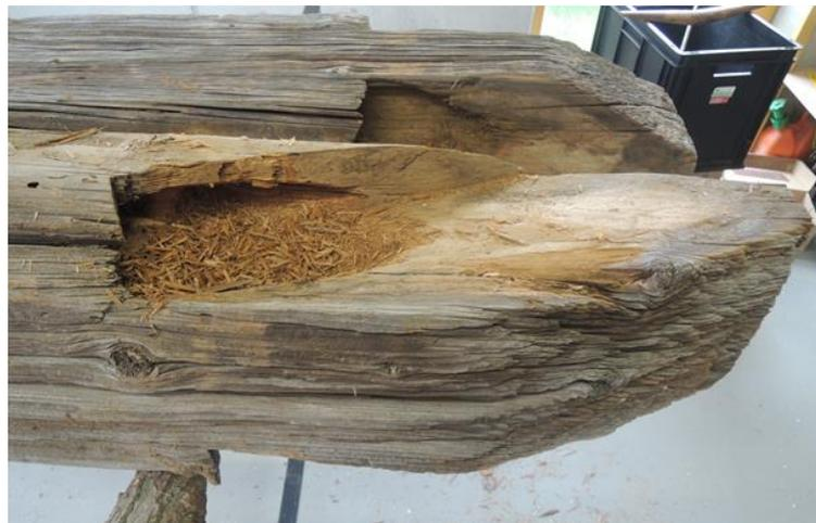
**Figure 23.** Damage to the beam (I2) in the location of the dovetail joint.
