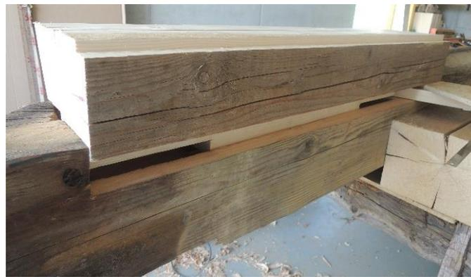
Figure 29. Formation of the insert and the gradual fitting.
