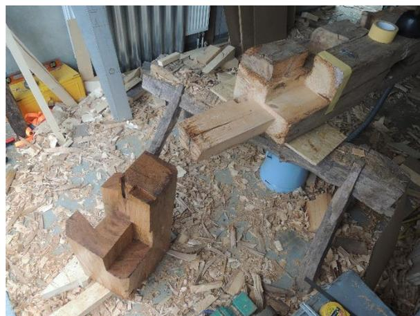
**Figure 8.** The new part before being inserted by a ledge joint.
