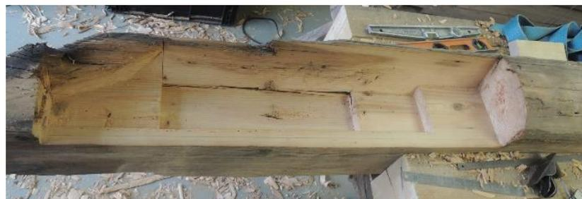
**Figure 27.** Finally cleaned part of the damaged beam.
