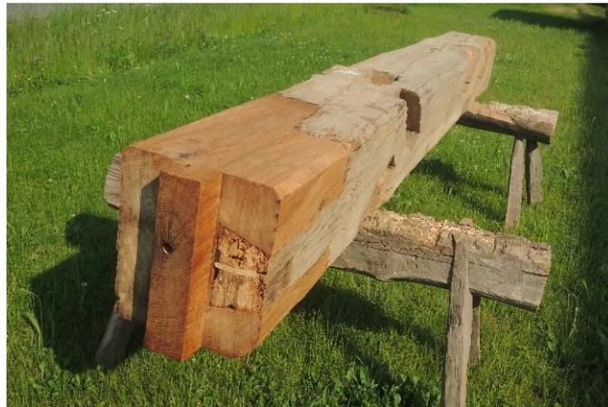
**Figure 9.** The bottom of the damaged beam (III) after the repair, including the ledge joint secured by a wedge placed in the drying check.
