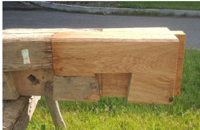
**Figure 10.** The bottom of the damaged beam (III) after the repair.
