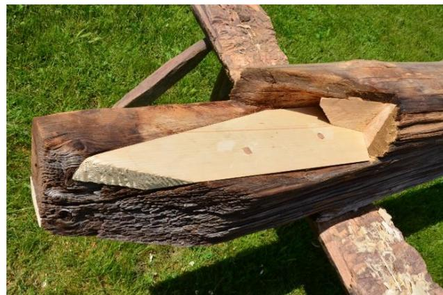
**Figure 19.** Dovetail joint of the damaged timber beam (H2) after the repair.
