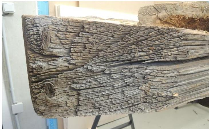
**Figure 15.** Detail of the damaged beam end before the repair, the end integrity ensured by the knot near the drying check.
