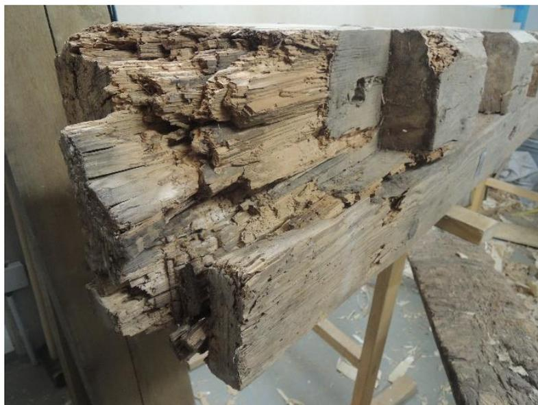
**Figure 2.** Damage to beam (III) at the bottom.
