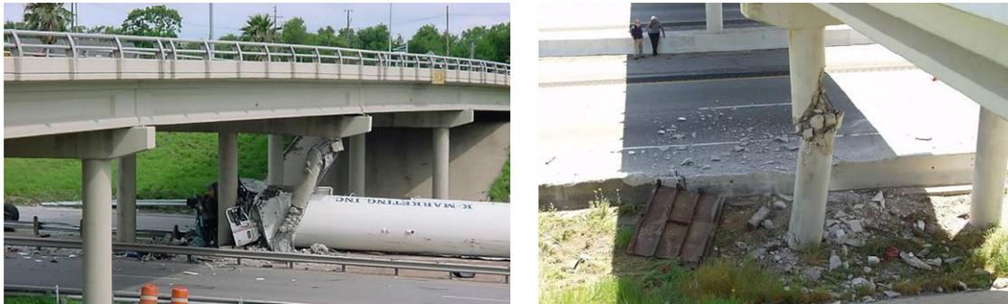
**Figure 1.** Bridge pier under vehicle collision [1].
