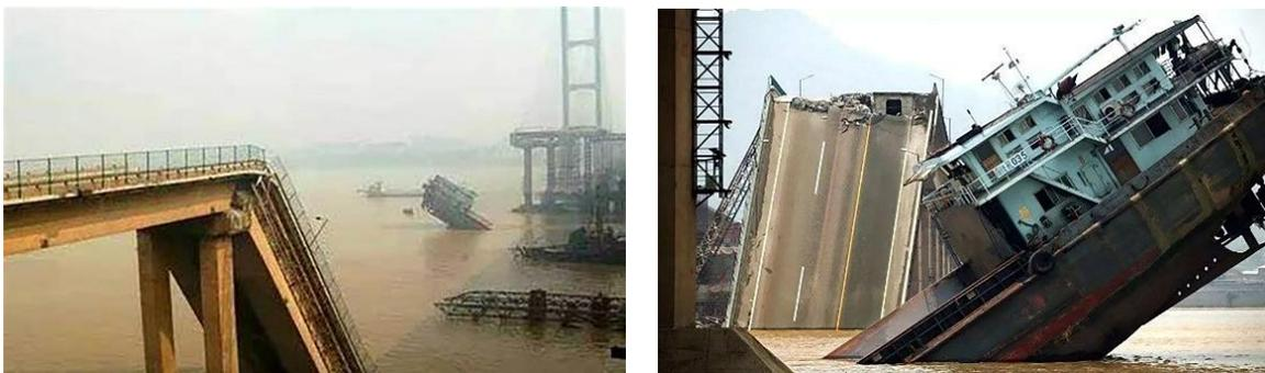
**Figure 2.** Bridge pier under vessel collision [2].
