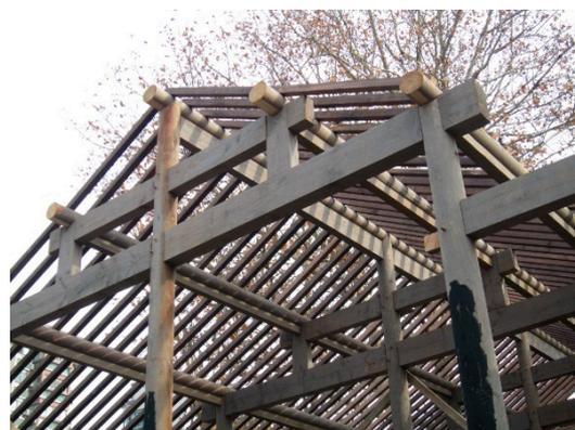
**Figure 2.** Straight mortise-tenon in timber frame.
