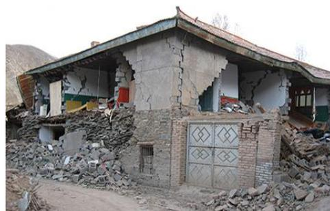
**Figure 1.** Damage phenomenon of concrete block masonry structure due to earthquake.
