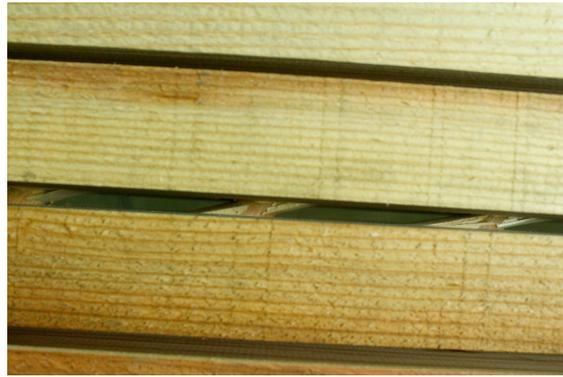
Figure 20. Split of wooden fibre on planks adjacent to dowels.
