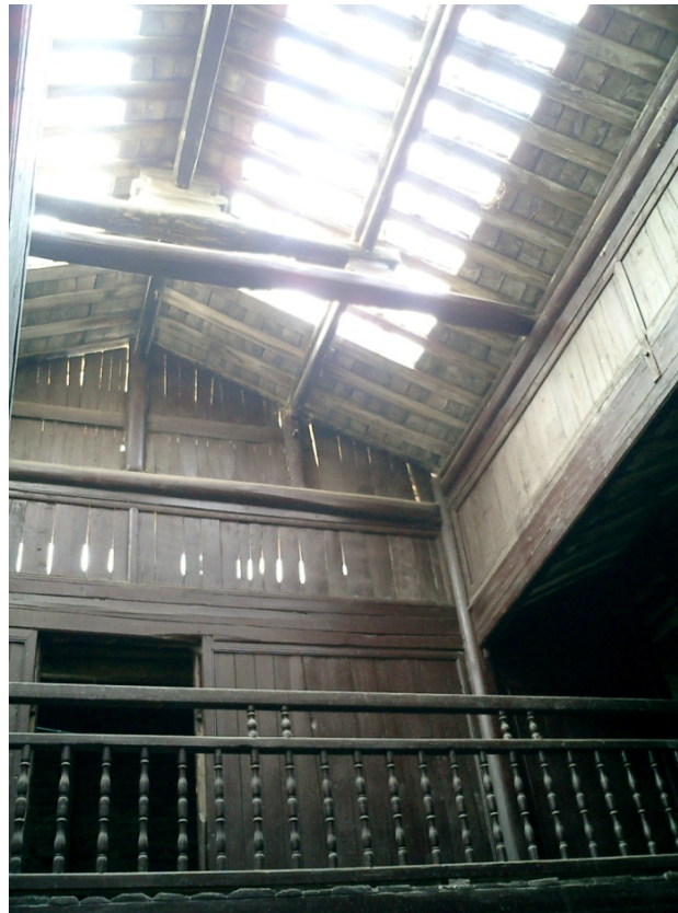
Figure 33. Ventilation of the roof.
