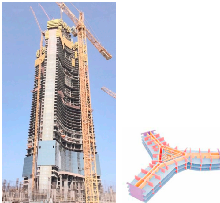
Figure 15. Jeddah Tower under construction (Courtesy of Jeddah Economic Company) and its structural layout (Courtesy of AS+GG & Thornton Tomasetti).
