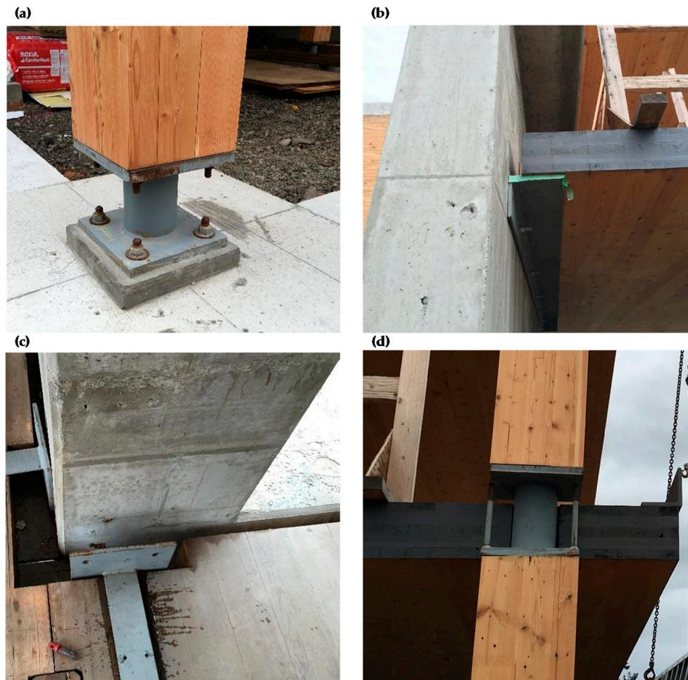
**Figure 2.** Joints: (a) Column-to-slab connections, (b) ledgers for floors, (c) steel drag strap connections for floors and (d) vertical connections for columns.
