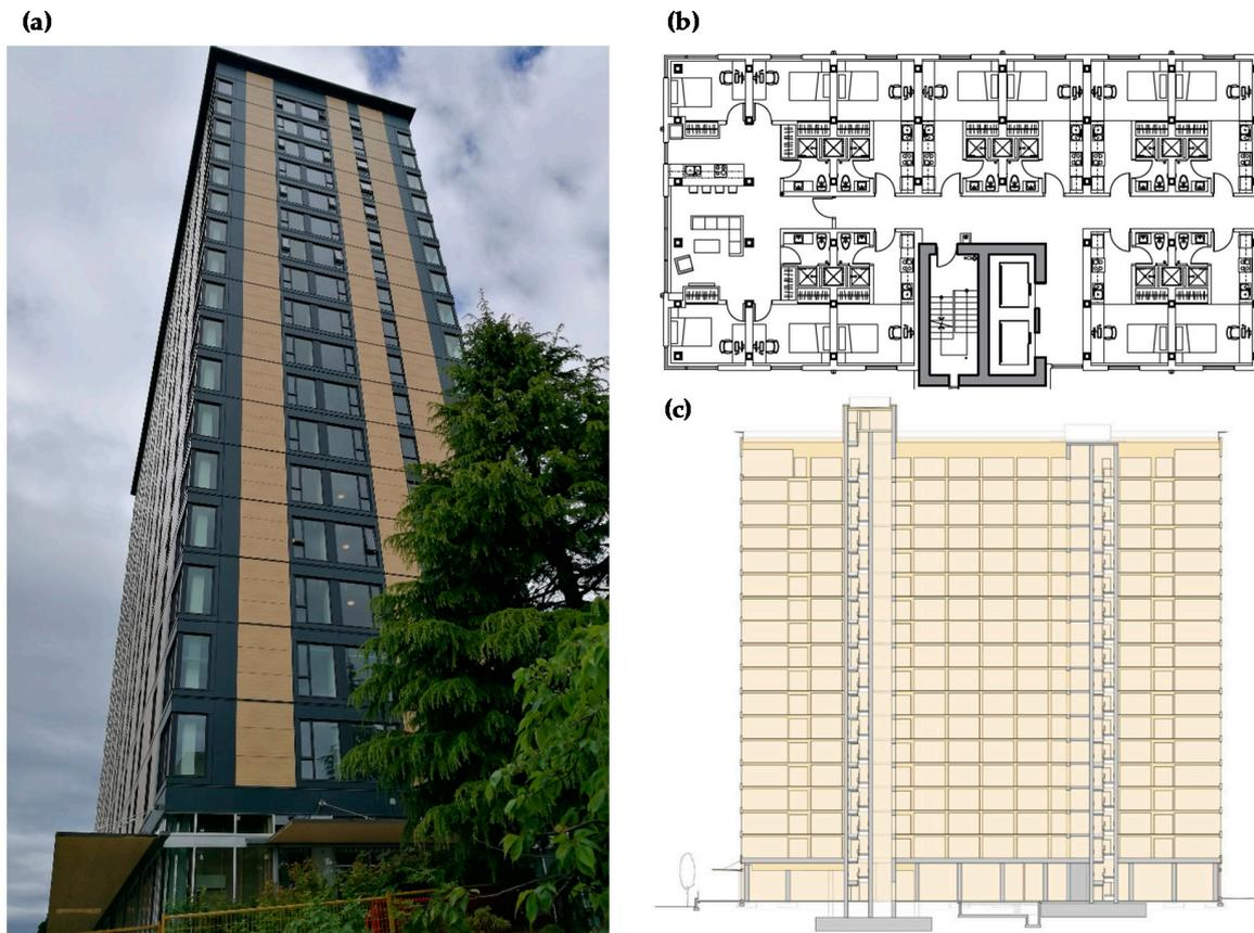
**Figure 1.** TWB: (a) building, (b) typical floor plan (partial section) and (c) longitudinal section (courtesy Acton Ostry Architects Inc., Vancouver, BC, Canada).
