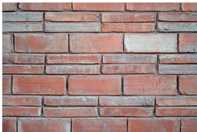
**Figure 18.** Special Lakhori bricks used for cladding the IHC building (Photo: Author).
