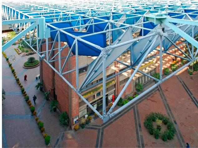
**Figure 19.** Sailcloth panels suspended from space frame to shade courtyards below (Photo: Author).
