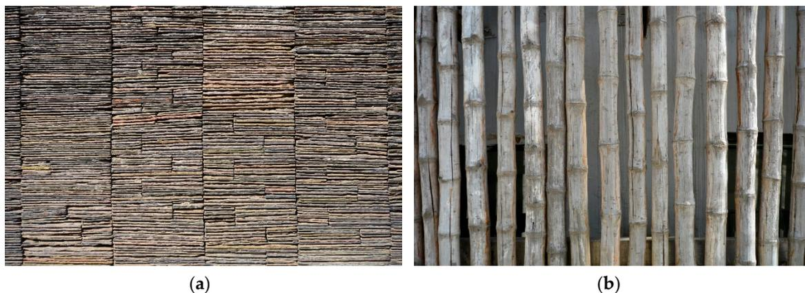
**Figure 35.** Cladding materials used in Dilli Haat Janakpuri: (a) Delhi Quartzite Stone and (b) bamboo (Photo: Author).
