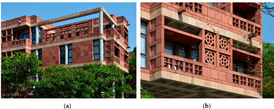
**Figure 10.** (a) Sandstone clad external skin delays heat transfer into the CIET building; (b) balconies and *jaali* screens protect the rooms of the CIET building from direct sun (Photos: Author).
