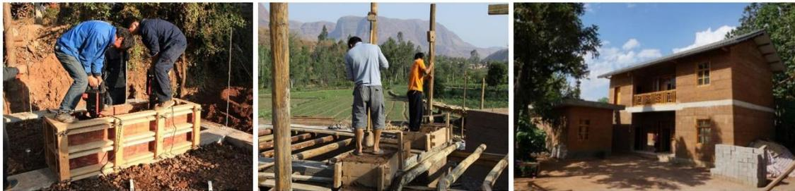
**Figure 7.** The reconstruction of Ma'anqiao Village in Sichuan Province takes advantage of the improved traditional rammed earth technique.
