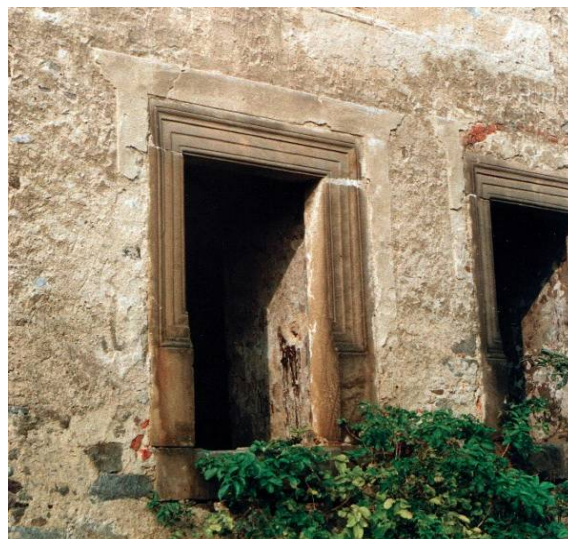
Figure 12. Window casings imitating stone detail on the facade of the manor house in Radzików. Photo author, 2003.
