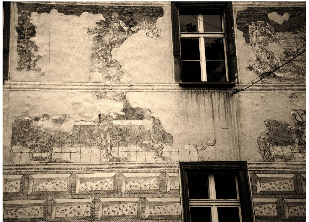
Figure 8. Remains of sgraffito decorations on the elevations of the castle in Prószków are united with a uniform background. Condition before renovation in 2011. Author's photo.
