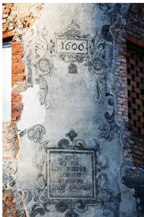
Figure 25. Sgraffito rollwork decorations on the walls of the palace in Broniszów (currently Zielona Góra Province). Photo by A. Legendziewicz, 2018.
