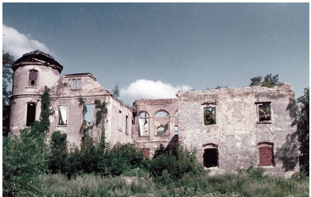
Figure 35. This Renaissance, single-body mansion in Zagrodno was expanded in the eighteenth century; its current condition is the result of building degradation that took place after 1945. Decorative sgraffiti were removed from the wall gable, the lower part of which is visible is on the right side of the photo. Author's photo, 2003.
