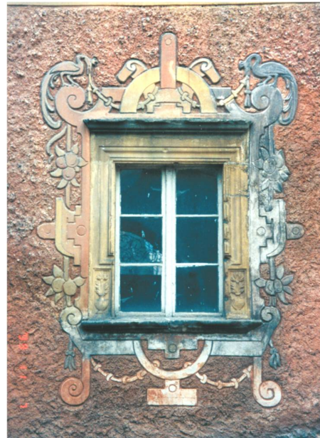
Figure 23. Sgraffito decorations around the windows with a rollwork ornament on the gatehouse of castle Gryf in Zagórze Śląskie. Author's photo, 2021.
