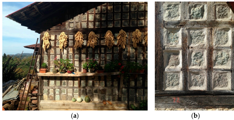
Figure 5. (a) Wooden facade with stone as filling material (Photographed by Ömer Faruk Bayram); (b) Relation of wood and stone in detail (Photographed by Ömer Faruk Bayram).
