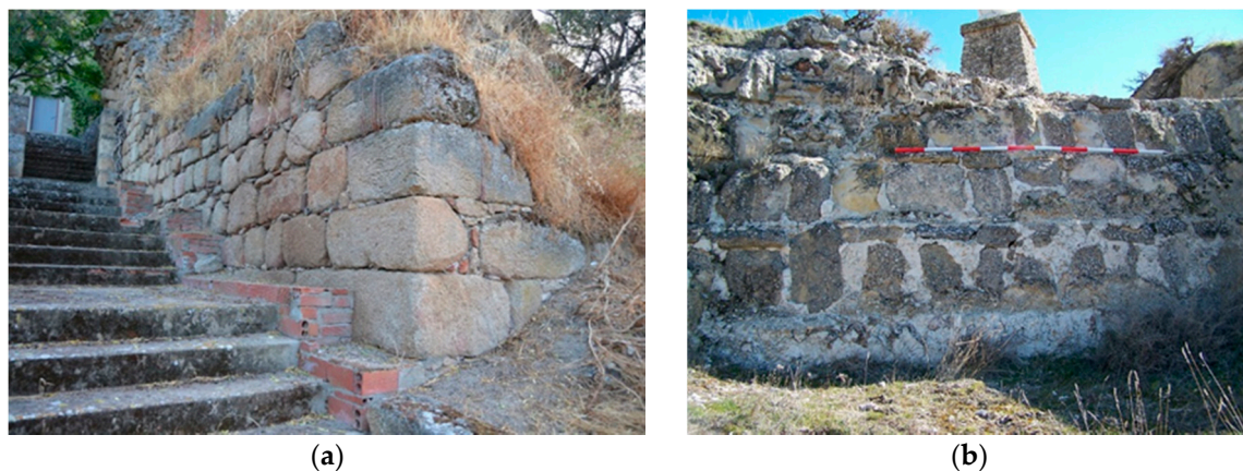
Figure 13. Irregular ashlar in (a) the alcázar of Alija (granite) and in (b) the alcázar of Huete (limestone) (photo: authors).
