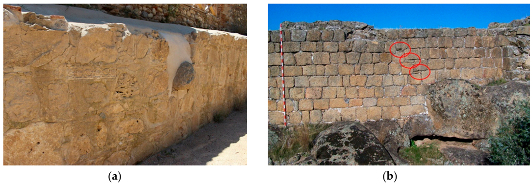
Figure 20. Chocks and level elements: (a) doorjamb or fine decorative late-antique plaque reused in the wall of Talamanca to level the row; (b) chocks in Vascos to level the row (photos: authors).
