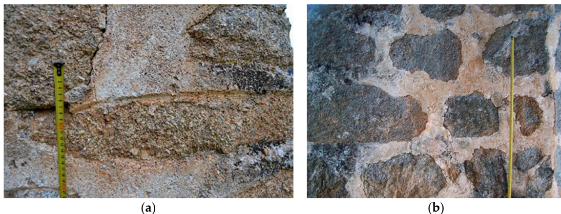
Figure 21. Final rendering of the walls in Vascos (a) with evidence of finishing tool (b) Covering space between stones in circular and irregular form (photos: authors).
