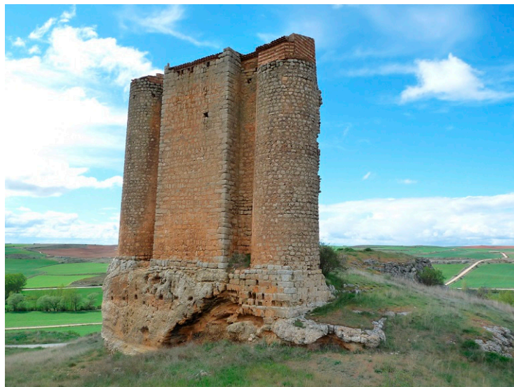
Figure 16. Ashlar masonry in the foundations of the castle of Soliedra (Soria) (photo: authors).
