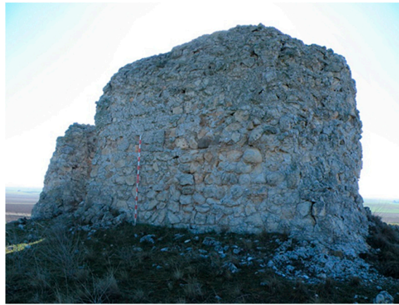
Figure 27. Tower of Fuente del Pez in Palomares del Campo; formworked stone masonry and gypsum-crusted external layer. (photo: authors).
