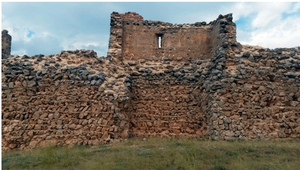
Figure 2. Detail of the inner part of the north wall in the castle of Gormaz. The construction shows that it was built quickly but systematically with a clearly organized design, assembled by skilled people. One row of poorly cut stones was not laid horizontally but appears slanted (this allows an arrangement of stone with different heights). Subsequently, a layer of lime mortar was poured on top of this layer order to achieve horizontal levels (photo: authors).
