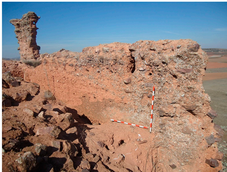
Figure 28. Eznavexor Castle. Concrete masonry preceding the Almohad phase (photo: authors).
