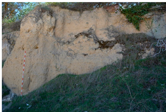
Figure 23. Huete city wall, in the area close to Las Tiendas; the wall and tower were built with rammed earth (photo: authors).
