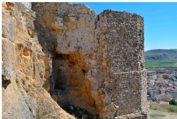
Figure 32. Vertical succession of masonries in the main tower of the alcazaba of Huete. The stone formworked masonry is laid over the Umayyad small sized ashlars and is anterior to the Christian phase (photo: authors).
