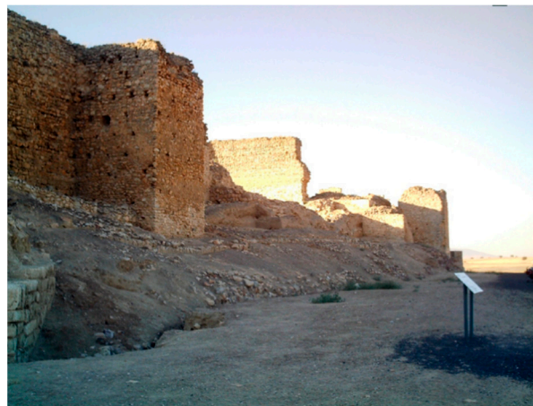
Figure 26. Lime and rubble masonry in the south wall of the madina of Calatrava la Vieja (photo: authors).
