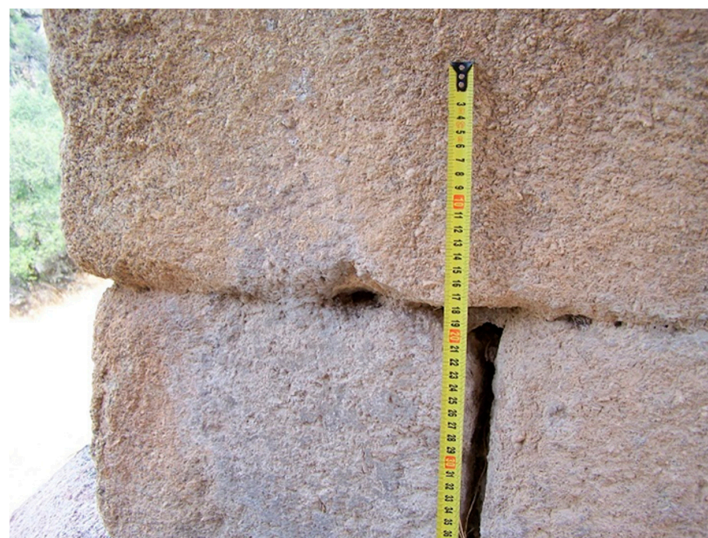
Figure 11. Use of a lever in Wicket Gate 1, Vascos (photo: authors).
