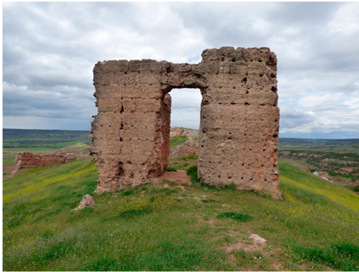
Figure 29. Alcaraz Castle. Towers in the middle of the fortress built with concrete masonry (photo: authors).
