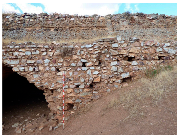
Figure 25. Formworked masonry in the castle of Salvatierra (photo: authors).
