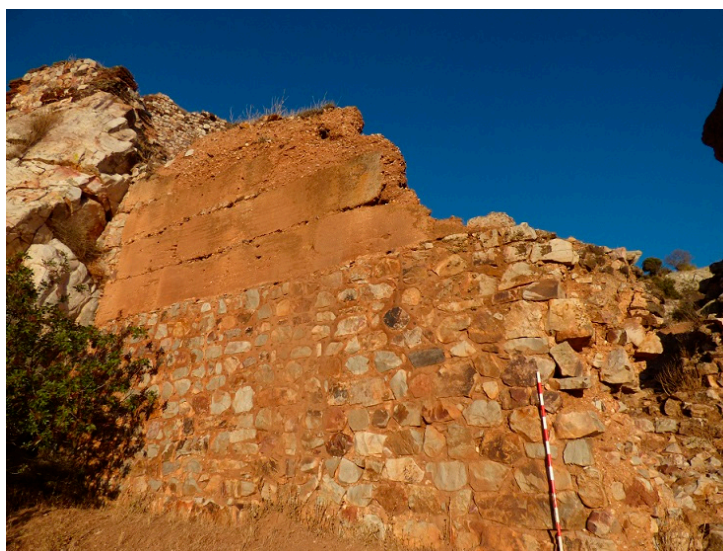
Figure 24. Lime-crusted rammed earth in the wall of the albacar in the castle of Salvatierra (photo: authors).
