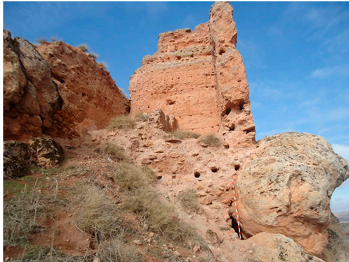
Figure 30. Tower of Gallo, in the castle of Montiel, as example of Almohad concrete masonry wall (photo: authors).
