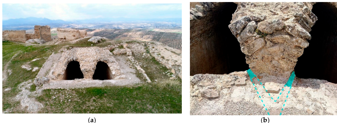
Figure 12. Cistern formed by two naves in the Alcazaba of Piñar. (a) View of the two naves cistern (b) Detail of the ceramic pipes at the joint of the vaults. Photographies by authors.
