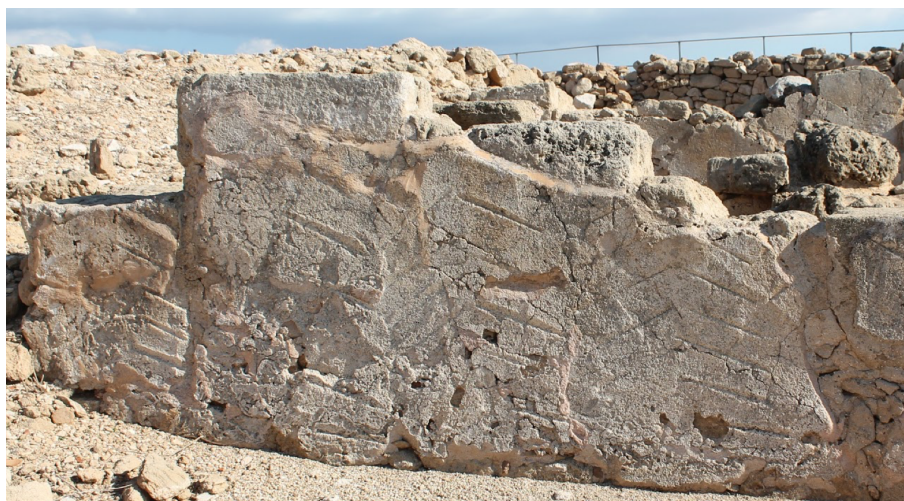
Figure 8. Herringbone incisions in the arriccio layer (base plaster layer) as preparation for subsequent plaster layers, from the House of Orpheus.
