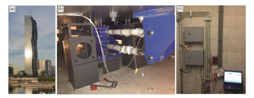
**Figure 18.** (a) Danube City Tower in Vienna, Austria; (b) MR-SVA of Danube City Tower with two controlled MR dampers and (c) two independent real-time controllers.
