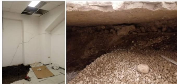
**Figure 10.** Cracks and siphoning below some buildings in Corso Trento e Trieste.
