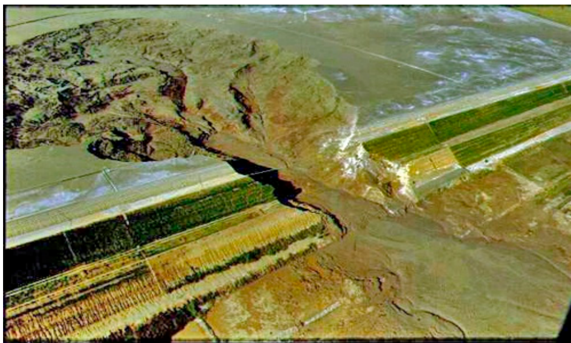
Figure A1. Aerial view of the Merriespruit tailings dam disaster. Approximate volume of the dam = 2.5 million cubic meters. Source: Tailings.info. Available online: http://www.tailings.info/casestudies/merriespruit.htm (accessed on 26 March 2016).
