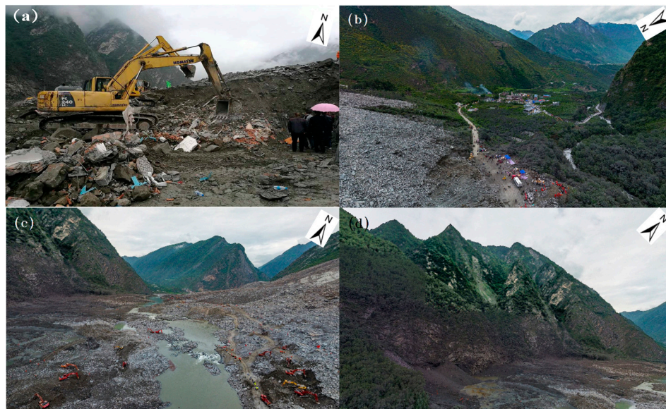
Figure 5. Close view of the landslide site: (a) Excavators involved in the rescue operation. (b) Houses not affected by the landslide, and the set-up of the rescue operation headquarter. (c) River being dredged after the landslide. (d) Debris of the landslide accumulated at the foot of the mountain.
