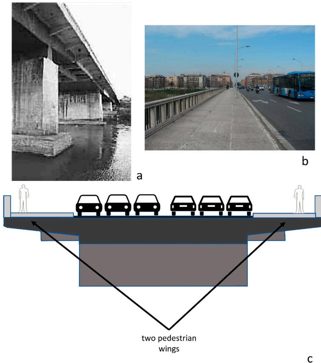
**Figure 5.** (a) The “winged” structure of the Marconi Bridge; (b) Note the difference between the sidewalk (covered by travertine) and the road (covered by the asphalt); (c) Schematic illustration of a section of the Marconi Bridge.
