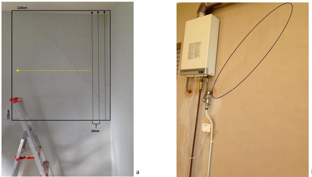
**Figure 3.** (a) The crack in the masonry and the dimension of the one-way grid; (b) shows a similar crack in the same wall in the balcony.
