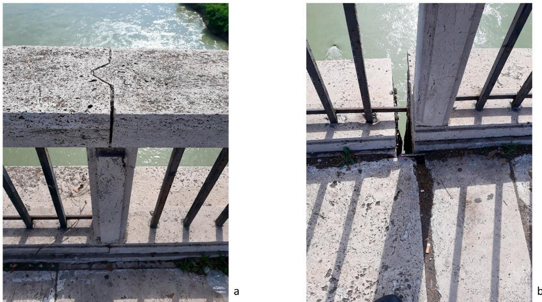
**Figure 6.** The visible detachments along the sidewalk of Marconi Bridge after Norcia 2016 earthquake (a,b).
