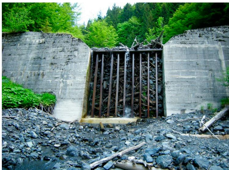
Figure 3. Seven-meter-high check dam in the middle section of the Suhelj torrent (modified from [25]).
