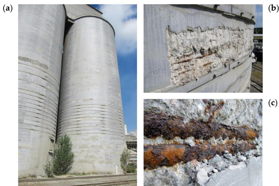
**Figure 9.** The tested structure of cylindrical silos for cement: (a) the outer shell surface of the silos; (b) corroded fragment of the perimeter wall with locally uncovered corroded reinforcement; and (c) very corroded steel rebars without concrete cover, directly exposed to atmospheric conditions.
