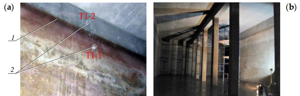
**Figure 5.** Photos from the inside of tested tanks for fresh water: (a) a fragment of the internal wall and floor slab of the tank: 1—smudge of water in the tank, 2—cylindrical concrete cores drilled below and above the line 1 that indicates water level in the tank; and (b) perimeter and internal walls, columns and beam from the reinforced concrete frame that supports the floor slab of the tank.
