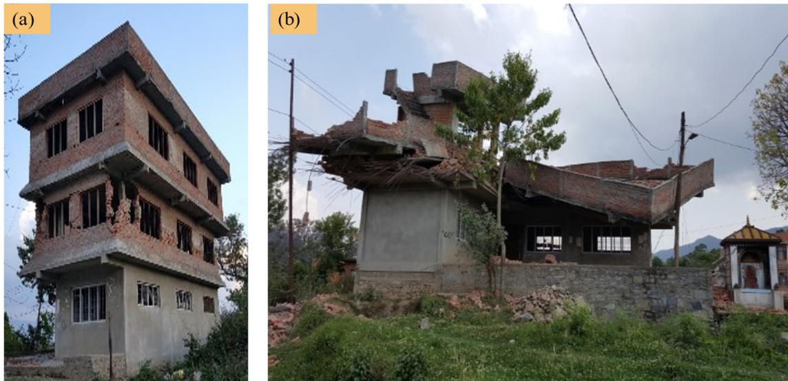
**Figure 1.** Damage to a residential building in Kathmandu by the 2015 Gorkha earthquake sequence: (a) after the 25 April mainshock; (b) after the 12 May aftershock (image courtesy of Krishna Devkota).
