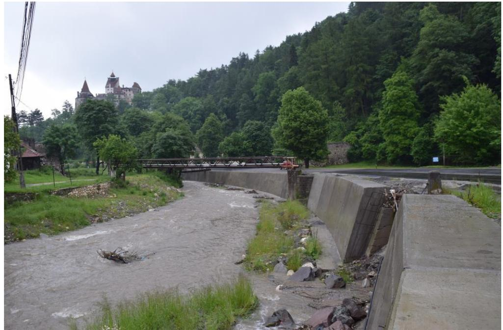
**Figure 20.** Turcu River in the Bran gorge sector (19 June 2021)—bank reinforcement straight with concrete wall for 144 m in length in front of DNE 73.
