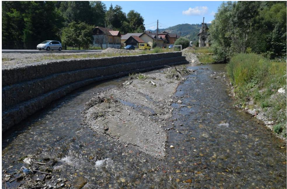
**Figure 18.** Turcu River at the confluence with the Shimon River (23 August 2020)—reinforcement of the right bank with gabions arranged in three steps over a length of 50 m at DNE 73.
