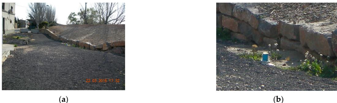
**Figure 7.** Settlement observed in the street after performing the PU resin injection treatment: (a) general view; (b) piezometric pipe (corresponding to borehole #2) used as a reference point; this borehole had a depth of 25 m and the pipe rested on firm ground. Note how the relative descent of the surrounding ground causes the pipe to protrude from the ground.
