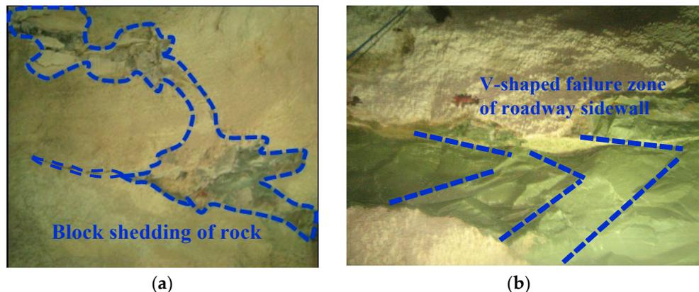
**Figure 3.** Failure characteristics of the roadway sidewall: (a) Block shedding; (b) Shape of destruction.
