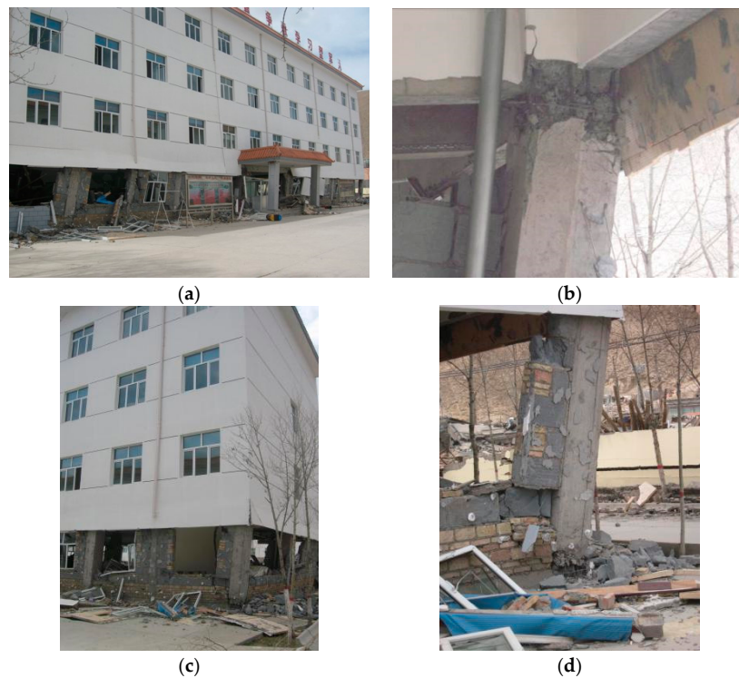
Figure 2. Seismic damage of the prototype building. (a) Bottom weak story mechanism; (b) 'Strong beam-weak column' mechanism; (c) Non-uniform damage along the height; (d) Damage at the bottom column root.
